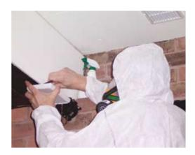
Externally, boarding around the roof line are common examples of cement based products which may contain asbestos if they were installed before the end of 1999.
