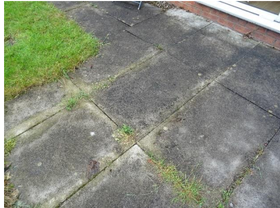
Rear paving – loose/uneven
