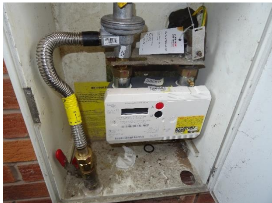
Gas meter and stop valve
