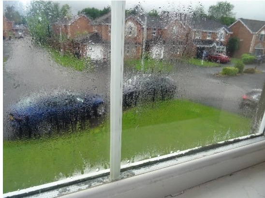
Misted/failed double glazing unit
