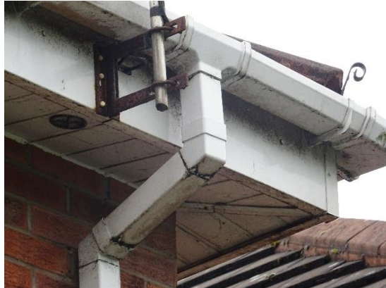
Leaking rainwater pipe joints
