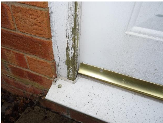
Weathered paint finishes
