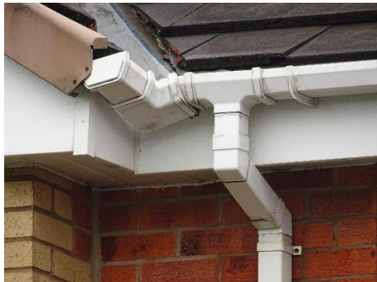
Loose guttering
