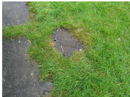
Inspection chamber
