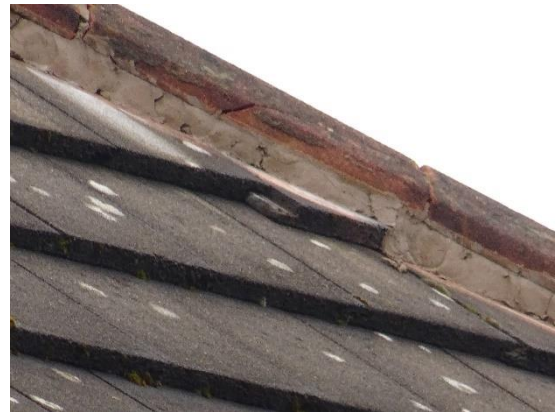
Damaged tiles
