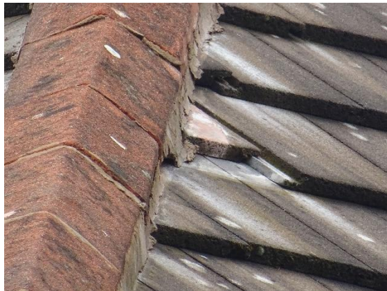
Damaged tiles
