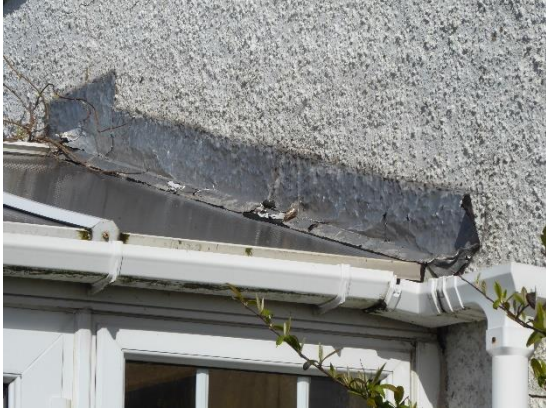
Temporary flashings
