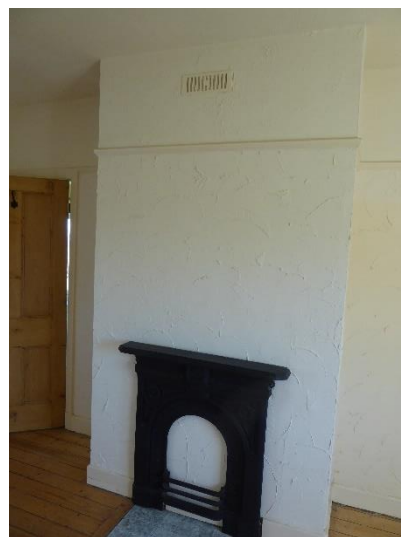
Chimney breast – large front bedroom
