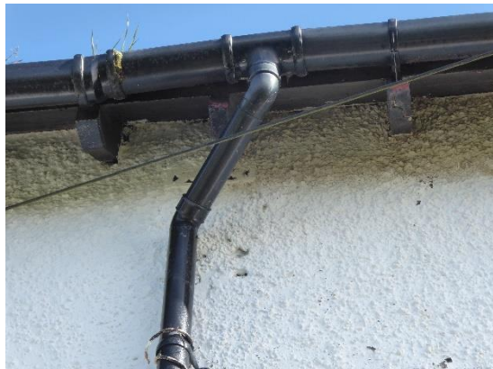
Leaking gutters
