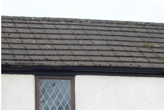
Front main roof
