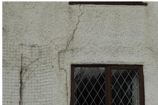
Render cracking
