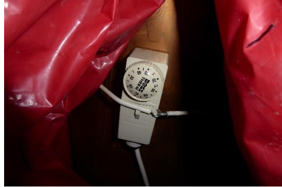
Cylinder thermostat
