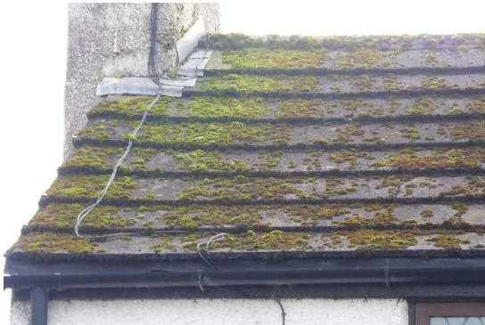
Rear main roof
