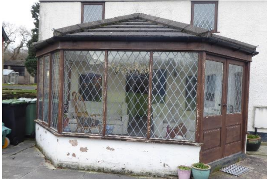
Sun Room - external
