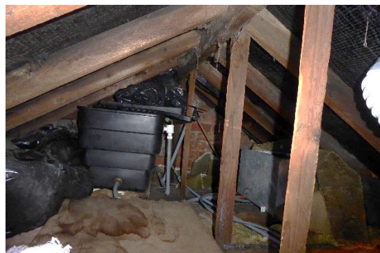
Main roof space/roof structure
