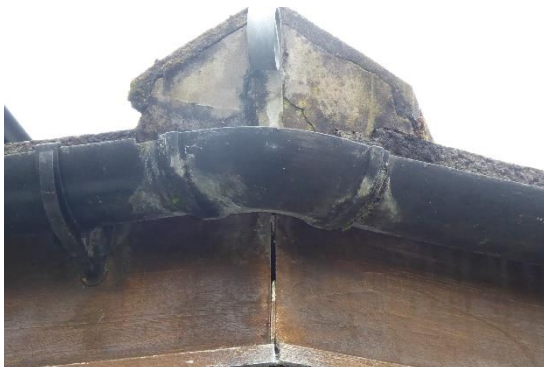
Leaking gutters
