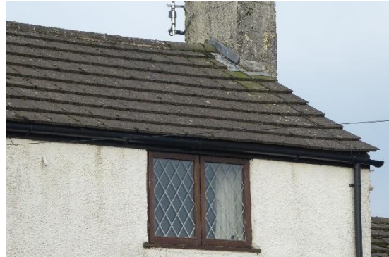
Front main roof
