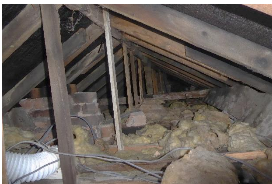
Main roof space/roof structure
