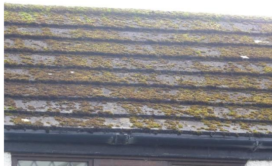
Rear main roof
