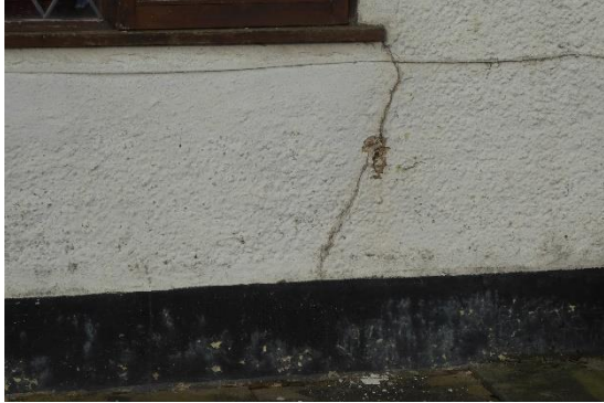
Render cracking
